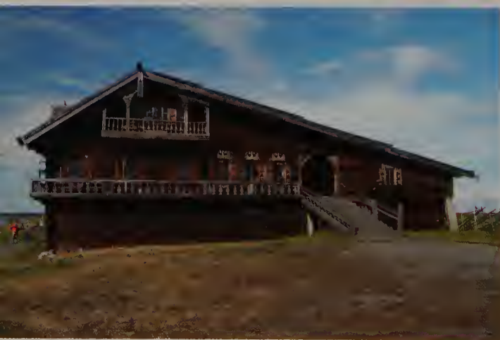
LEFT This is an example of a common northern form of izba , the two-story koshel (basket house) in which the living quarters and the agricultural spaces are integrated into one building.
