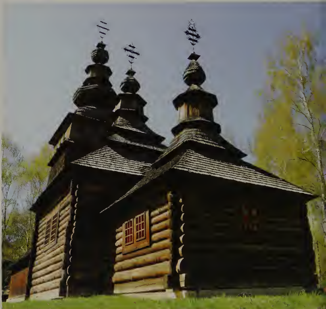
ABOVE The distinctive three-tier structure of a Carpathian Lemko church, built entirely of intersecting wood logs with wood shingle roofs topped by spires and cupolas.
