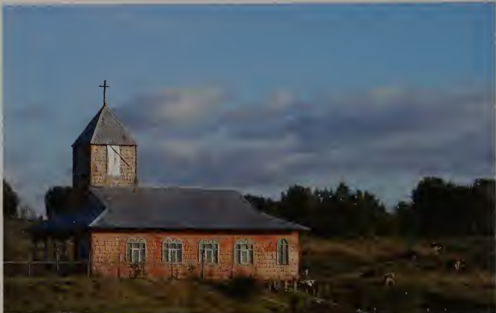
ABOVE This shows the typical style of wood church building on the island of Chiloé off the coast of Chile, with its rectangular basilica divided into three naves by wood columns, a roofed portico, a main roof of wood shingles, and a symmetrical tower at one end.
