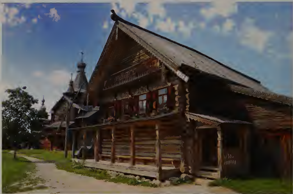
ABOVE An elegant and sizable example of a Russian izba , a wood house with a small attached barn, built of logs with interlocking corners and a sloping wood shingle roof. The posts of the wood portico, eaves, window frames, and doors are carved and embellished (see detail left).
