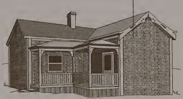
Horizontally laid bottles cemented to form walls
